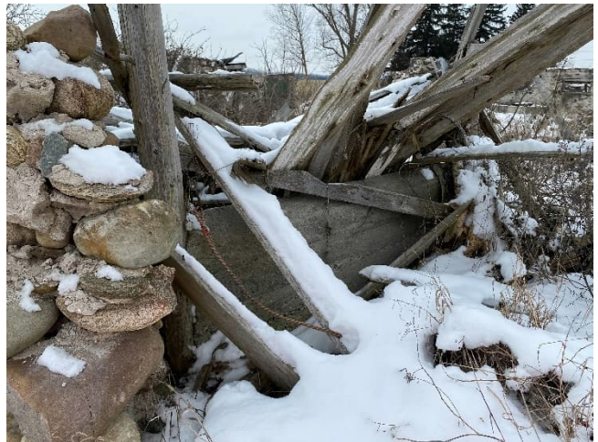
Plate 26: Wood beams and planks
