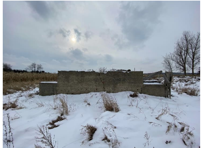
Plate 20: East end wall outbuilding ruins
