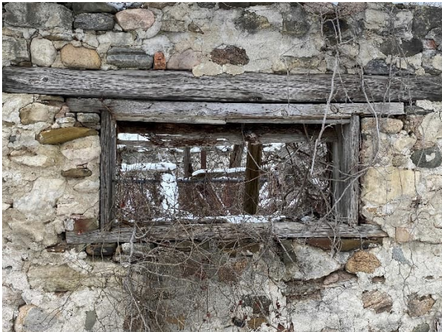
Plate 15: Wood lintel and window frame
