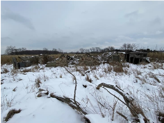
Plate 17: North elevation of outbuilding ruins
