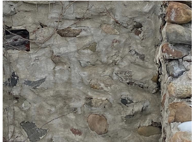
Plate 14: Parging on fieldstone wall
