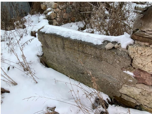
Plate 21: Cast-in-place concrete wall
