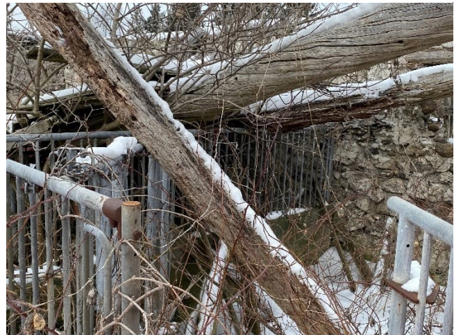
Plate 16: Remnant wood floor beams
