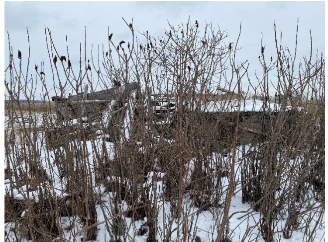
Plate 18: West end wall of outbuilding ruins
